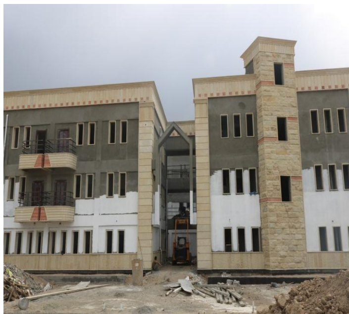
Figure.9 External Finishing Progress of the Projects
